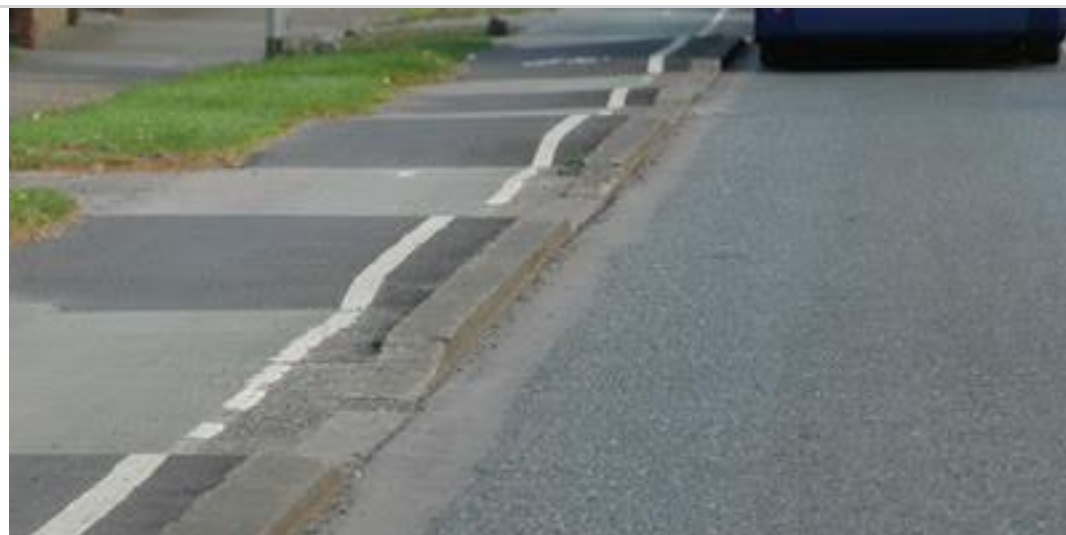
2. Driveways may not influence the level of the sidewalk or cycle path.
